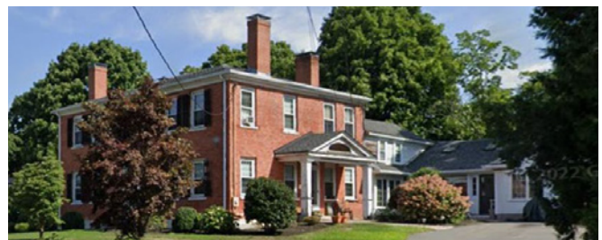
Elijah Fiske house, built ca 1801, at 457 Lincoln St. (Google street view, 2022)
