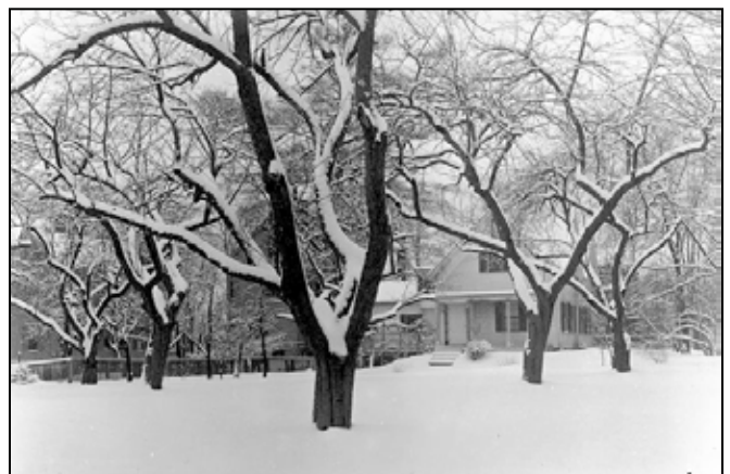
Stephen B. Cram's orchard, Crescent Street, corner of Moody Street (now a gas station)
